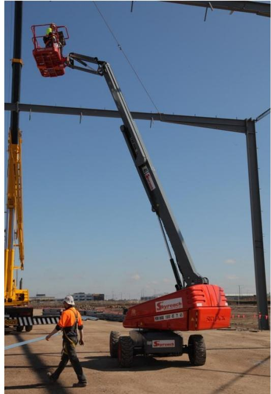
A significant benefit of the Skyjack SJ45T is the 4WD drive, all terrain system. The front axle has a limited slip differential, while the rear axle utilises a 'no-spin' differential. A capability to move up a 45° incline ensures that this unit is able to operate on the most difficult work sites.
